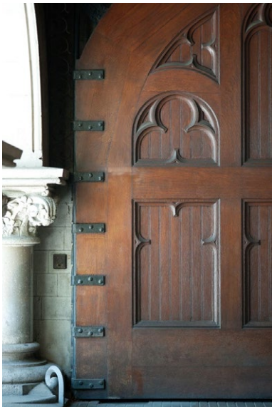
Figure 8. Main street door detail of the Casa Vidua Marfà
