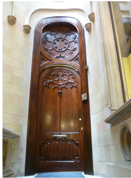
Figure 7. Access concave door of the Casa Vidua Marfà
