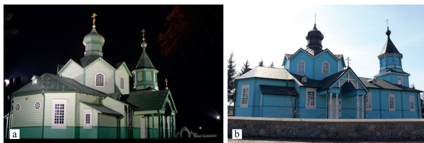
Figure 6. A view of the parish church of the Exaltation of the Holy Cross in Narew: a) before renovation in 2019, author: unknown (source: https://www.portals.narew.gmina.pl/parafie/98-parafia-prawoslawna-w-narwi , access: 2nd May 2023); b) March 2023, author: Katarzyna Woszczenko.
