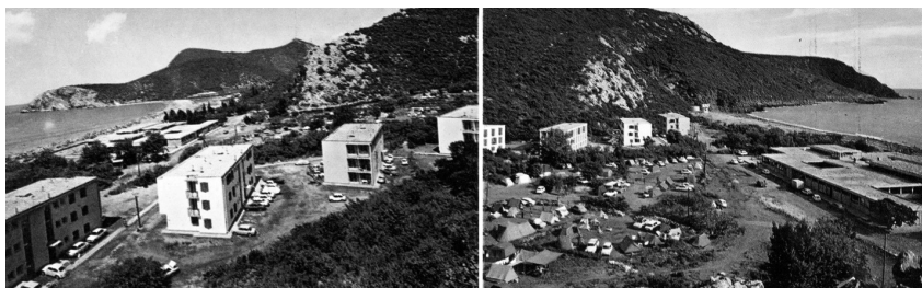
Fig. 1. Tourist complex and summer camp in Čanj – Bar Municipality, from the 1970s.
